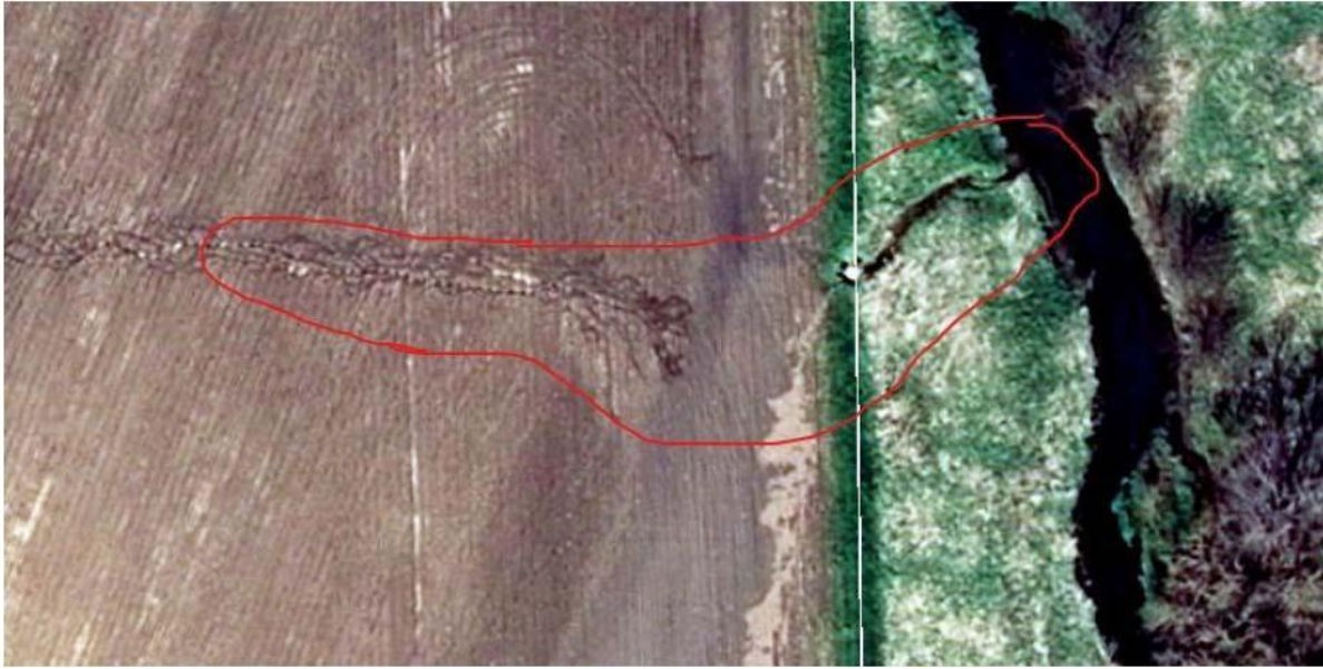
Parcel 11: Significant erosion at the edge of a corn/soy field in the Lake Springfield watershed has runoff leaving the field in channel flow, eroding a tight channel through the buffered area and dumping directly into a nearby waterway
